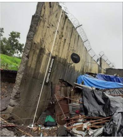
property from informal settlements was the purpose of the wall, a mesh wire fence mounted on a retaining wall would have served both purposes (allowing road construction as well as protecting the property).
